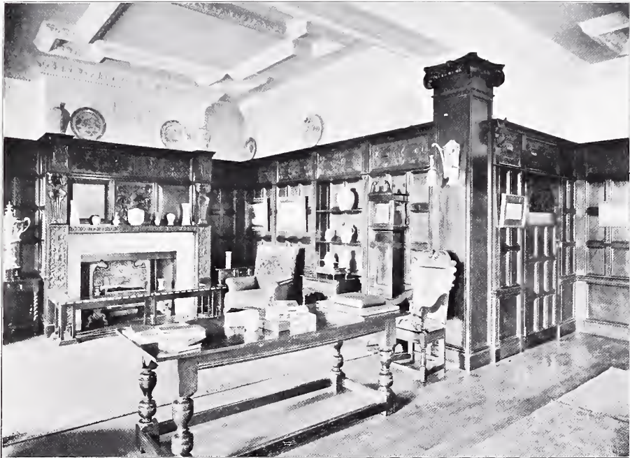
Alcove in Billiard Room.
